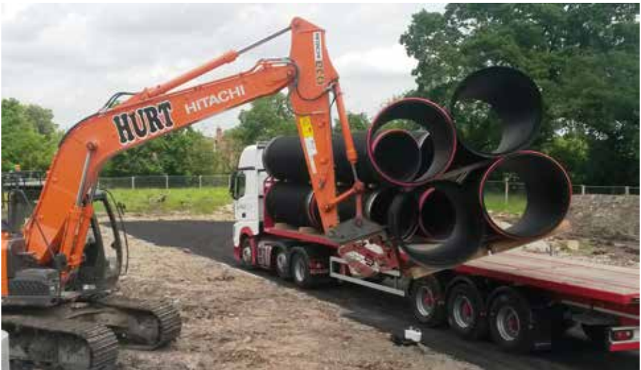
Figure 2: Pipes being unloaded utilising extended forks.
