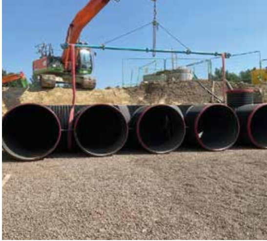
Figure 24: Installation of a manifold utilising a lifting beam.
