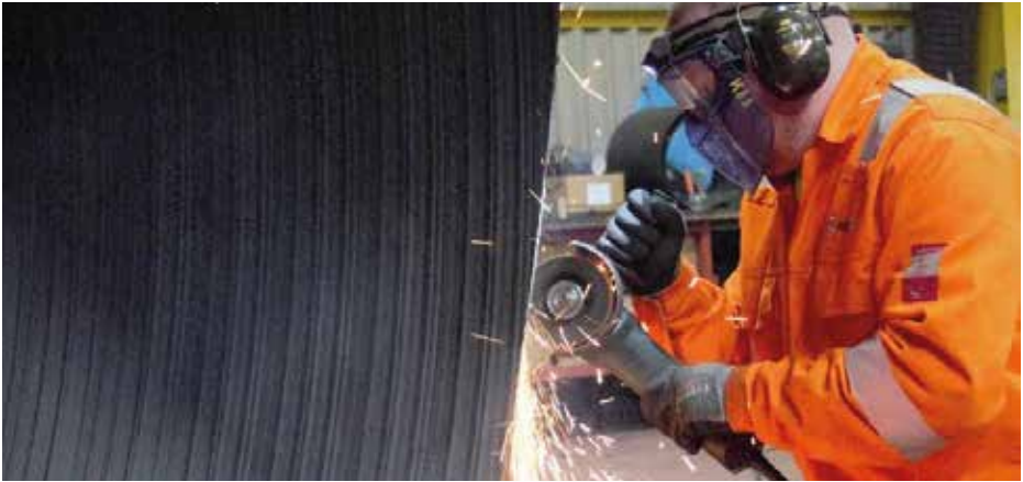
Figure 35: Cutting a CSR pipe using 125mm angle grinder.
