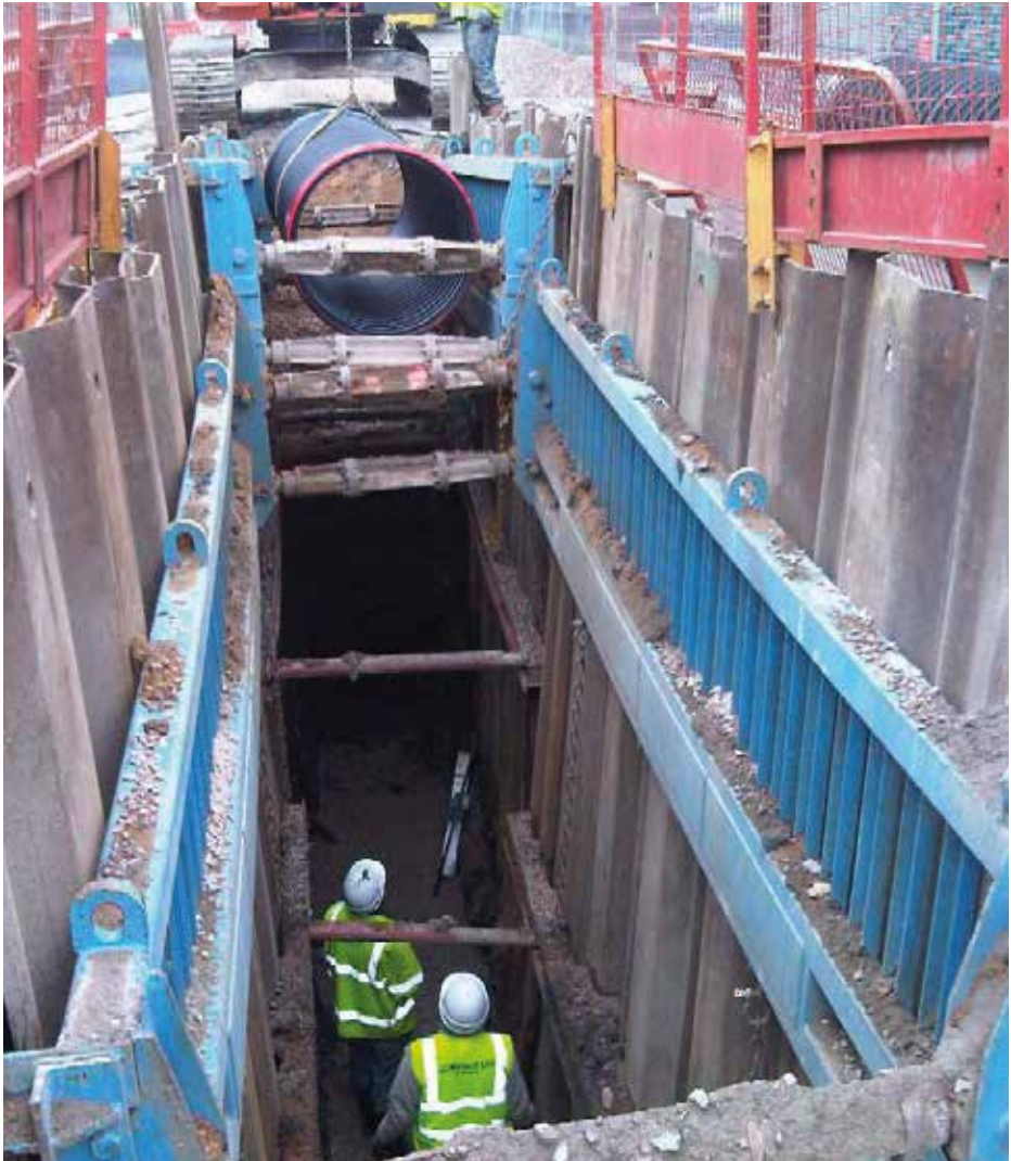
Figure 10: Handling CSR pipe during installation.
