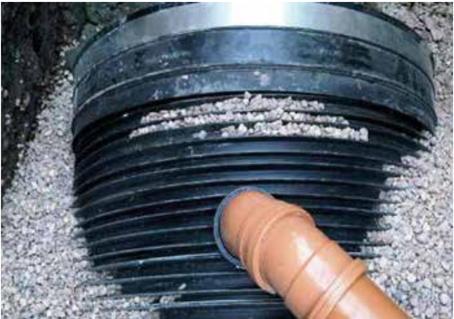
Figure 21: Picture of a completed gully connection.
