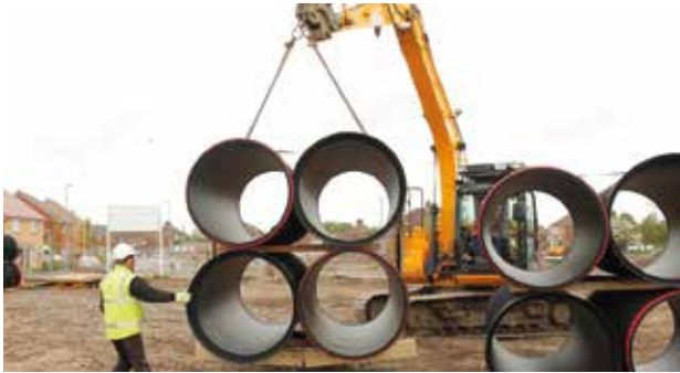
Figure 5: Moving CSR pipes around site.
