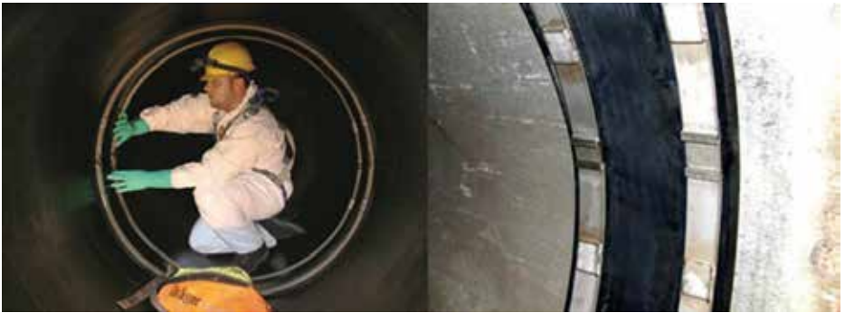
Figure 16: Internal repair mechanical coupling.
