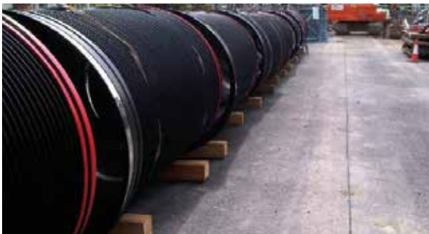
Figure 6: CSR pipe storage on highway ensuring pipes are chocked.
