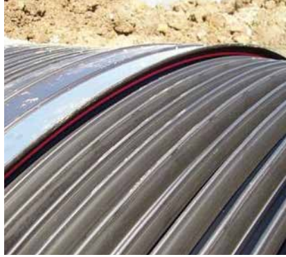
Figure 12 CSR correctly jointed socket/spigot.
