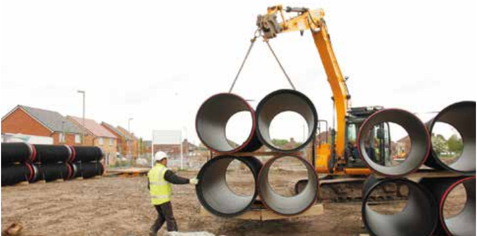
Figure 4: Unloading CSR pipes in packs utilising lifting straps.
