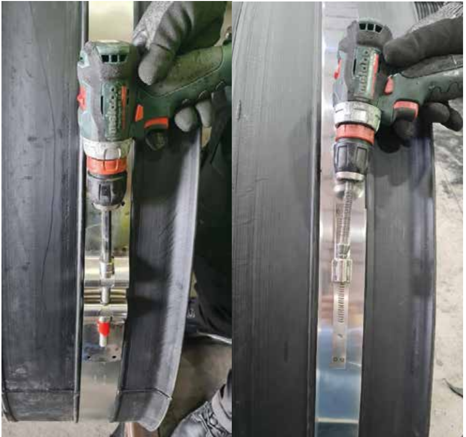
Figure 13: Tightening creep band using a cordless drill and either 8mm 100mm long hex attachment (left) or an M10 with 8mm socket head cap for worm drive (right).
