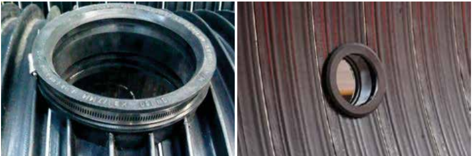
Figure 20: Installation of the LTC.
