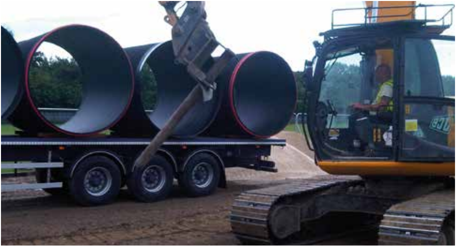
Figure 3: Unloading utilising a pole attachment.
