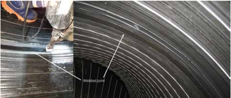
Figure 17: Extrusion Welding.
