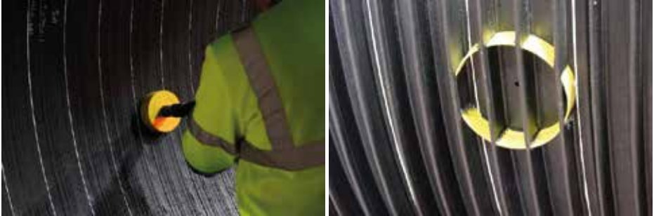
Figure 19: Drilling CSR pipe internally for gully connections.
